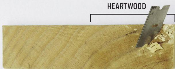
Decay in heartwood LOSP treated
